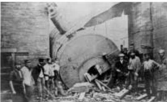
Figure 1. Aftermath of boiler explosion, probably caused by caustic cracking. Picture courtesy of IMechE.
